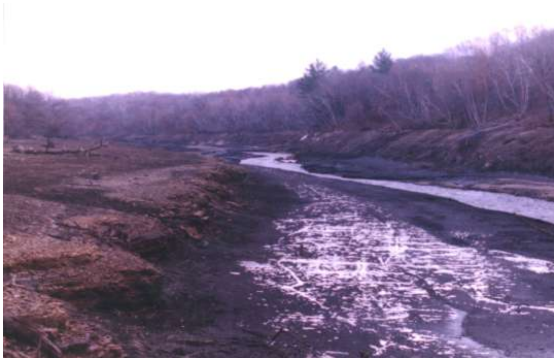
Former impoundment of Mounds Dam, 1 week after removal
