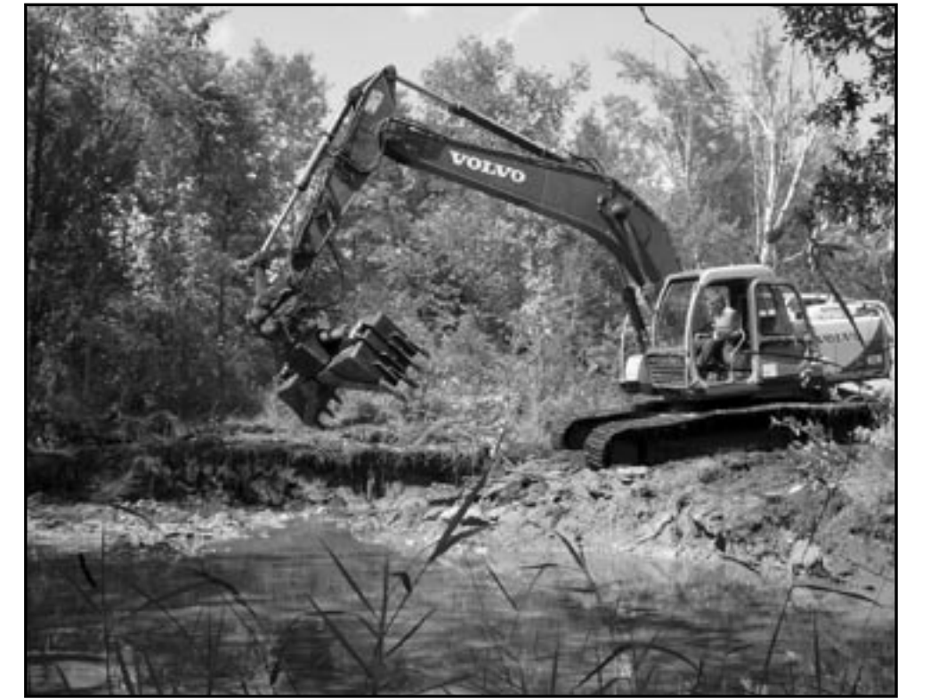
Spitzer Dam was no match for this backhoe - and restoration begins.
