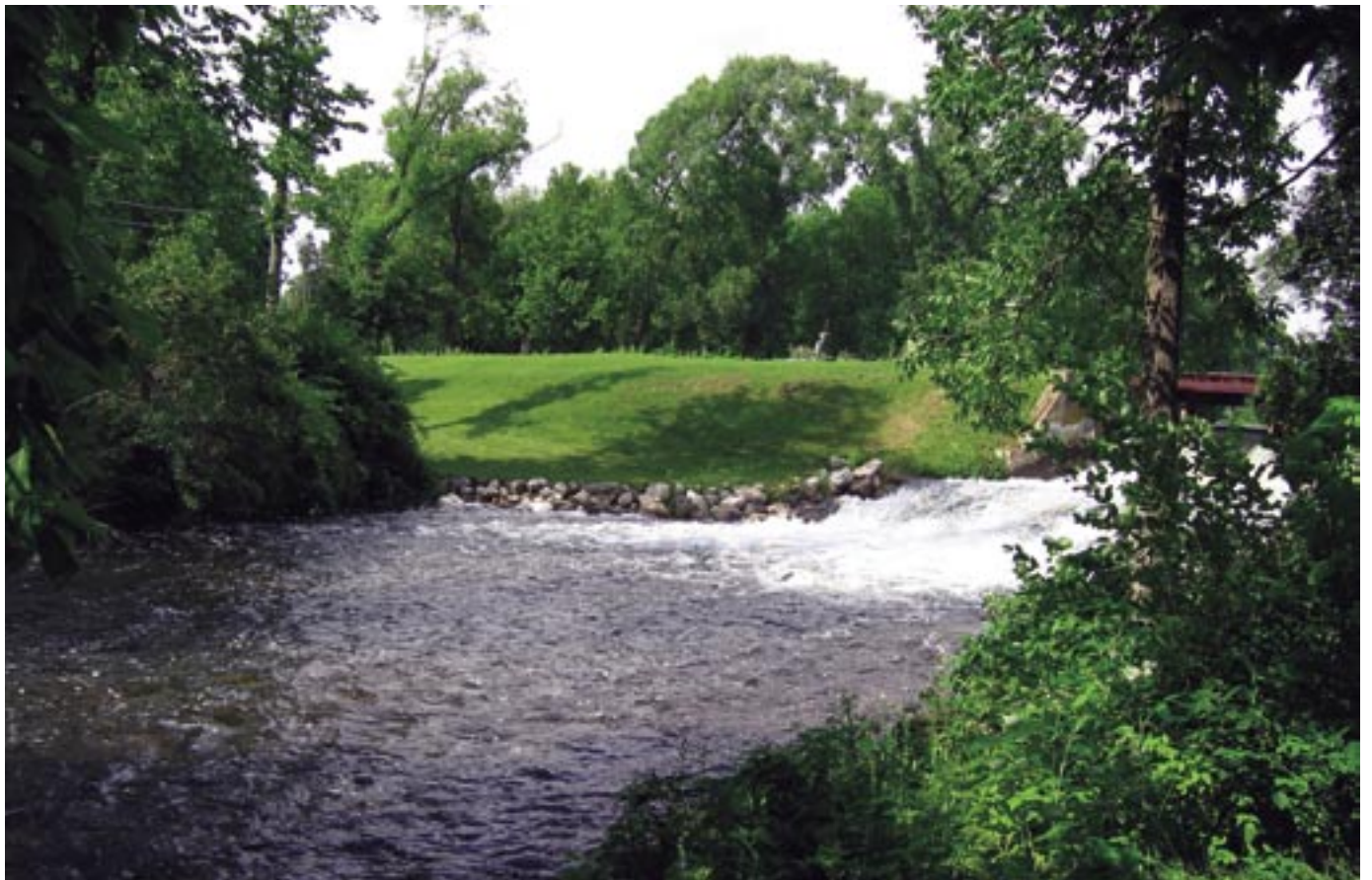
The Bark River downstream from the Nemahbin Roller Mill Dam, constructed in 1839. River Alliance photo
