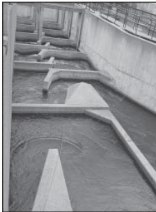
Fish ladders at the Bonneville Dam in Oregon. Salmon and other species wind their way upstream and around the dam. Photo: Michael Lavitschke
