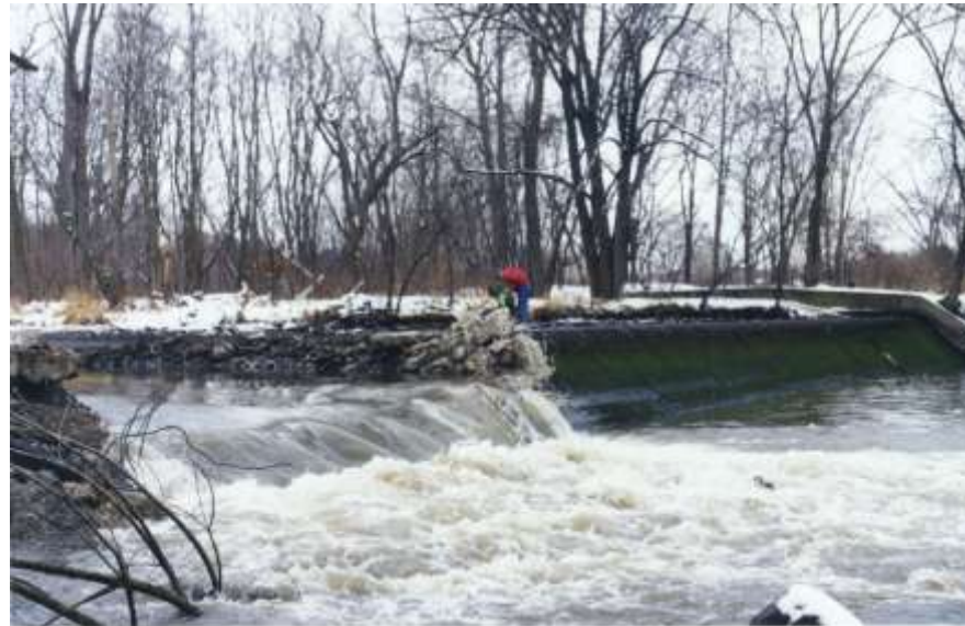
Waterworks Dam removal, Winter 97-98
